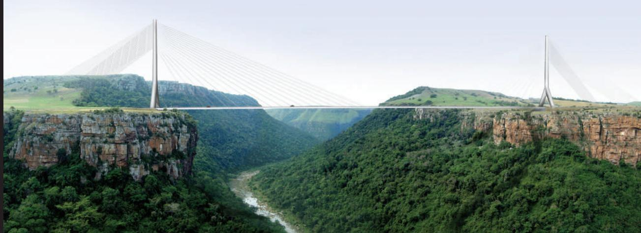
Surbana Jurong (**No. 24**) unit SMEC is providing design services on the Msikaba Bridge in South Africa, with its 530-m composite concrete and steel deck to be supported at both ends by 17 pairs of both mainstay and backstay cables anchored into 127-m-tall reinforced concrete pylons. When complete, the bridge will be both the longest and highest single-span cable-stayed bridge in Africa, the firm says. ■
